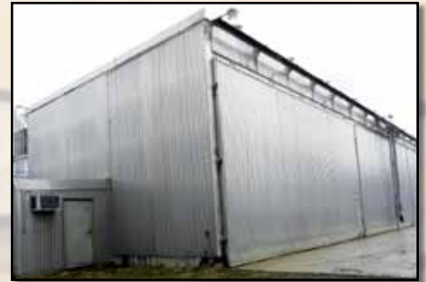
2000 NARDI 150,000 Board-Foot Cap. Timber Drying Kiln, (3) bays @ 50,000 each w/Leonardi controls
